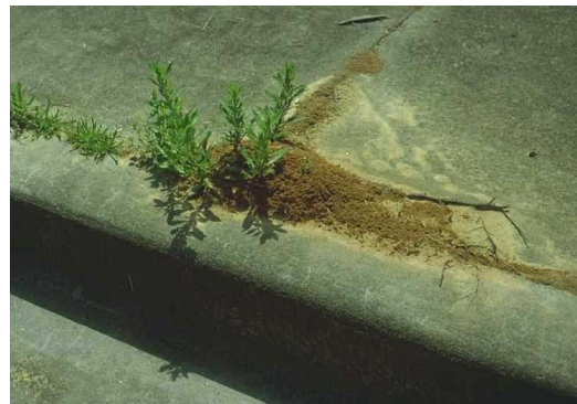
Fire ant mound in sidewalk.
